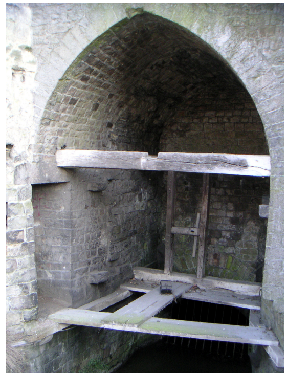
The water gate in the Dodenne tower, on the east side of Valenciennes, is the only survivor of the 16 th century fortifications
