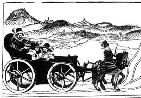
4.3 Measurement by coach wheel, from Paul Pinzing, Methodus geometrica , 1598.
